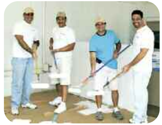
ABOVE: Trading their banking duties for paint brushes, Scotiabank employees (from left) Ricardo Ortiz, Milvio Medrano, Carlos Rosa and Carlos Soto created a bright new space for a school computer room in San Juan, Puerto Rico.
