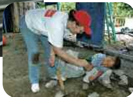
THIS PAGE: Over two days in October, Scotiabankers helped a family in Tepecoyo, El Salvador realize the dream of a solid new home as part of the A Roof for My Country program.
